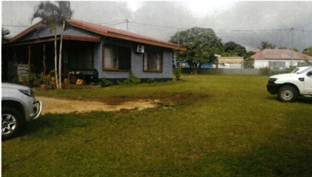
Photo 1: NEW BUILDING SITE - IN FRON OF EXISTING OFFICE
